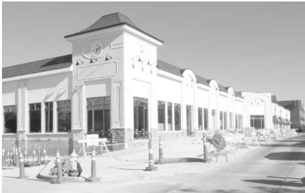
Oakwood's new retail building at Far Hills and Orchard Ave., which reflects a typical new urbanism design and scale.
